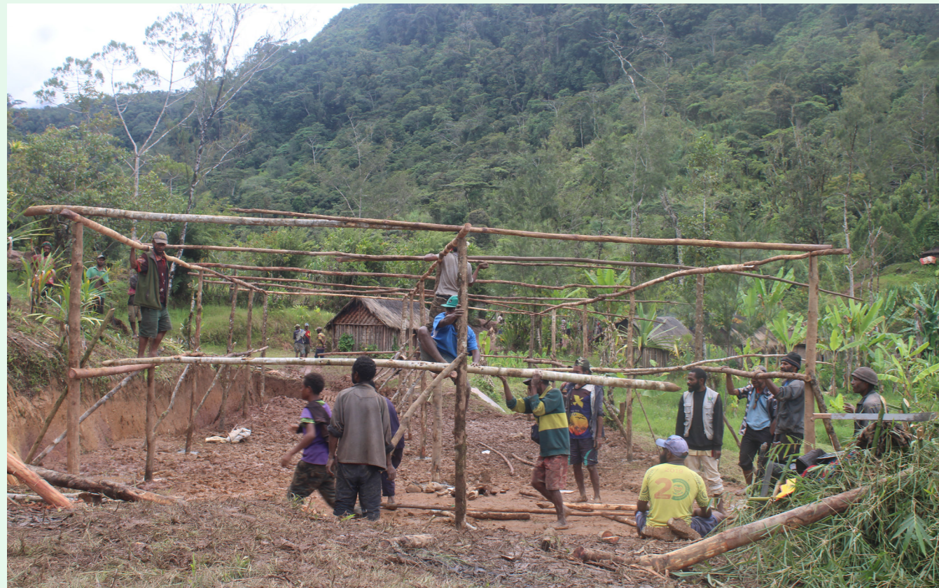
Nursery construction at the project site © WCS Papua New Guinea
